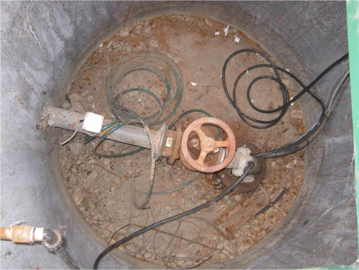
Photo 2: Bore 2 headworks
